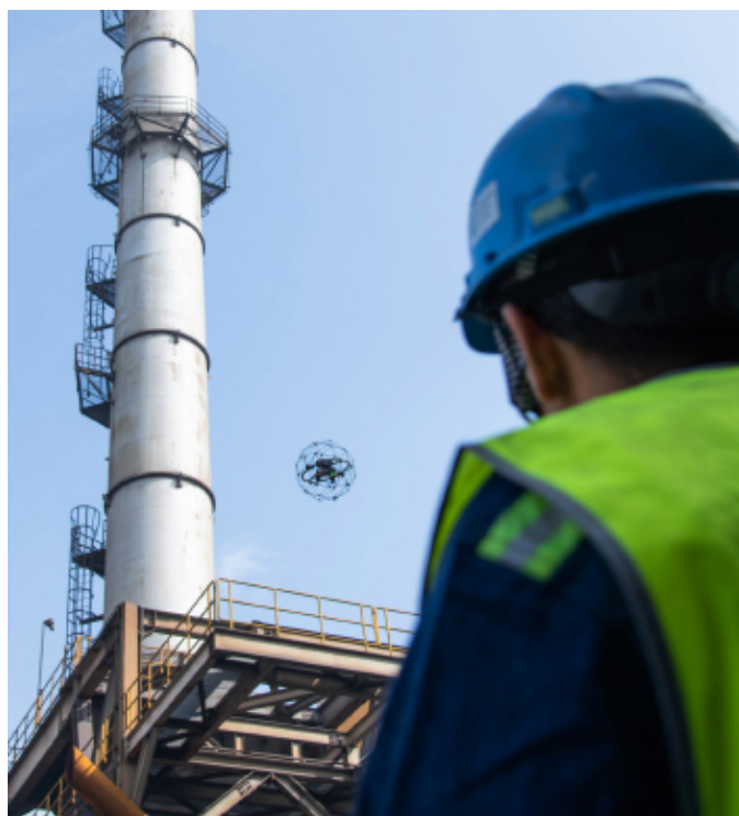
INSPECTION AT HEIGHT. The drone technology replaces manual inspection, thus eliminating complex tasks.
